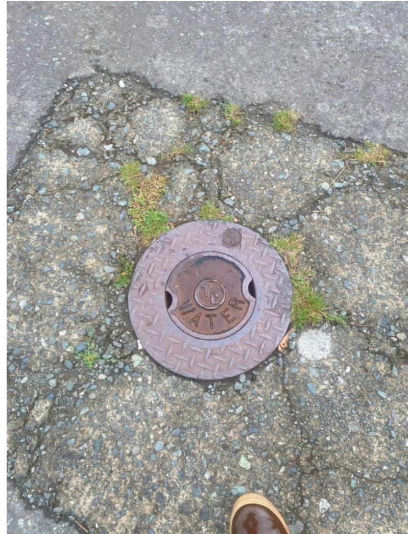
Photo 12. August 18 th , 2025. Municipal watermain on the ERT Road across from the SWDP headwall where drainage from the headwall is believed to be directed to.
